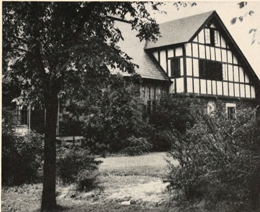
James Gamble Nippert Memorial Lodge, 2707 Clifton Avenue, Home of Ohio Epsilon at the University of Cincinnati, since 1925.
