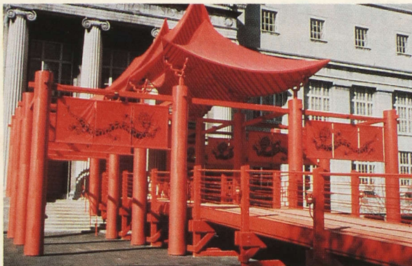
Main Entrance Ramp
