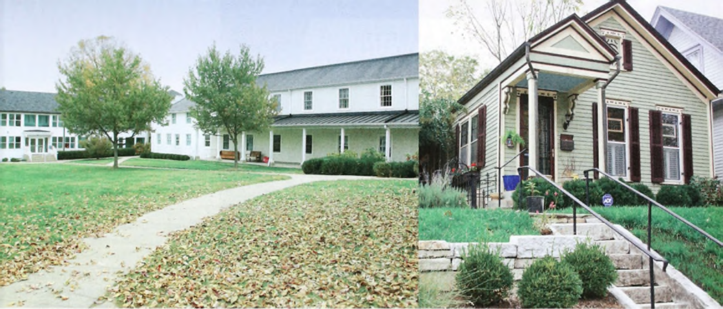
Left: Some of the buildings at the Stuart Home School, formerly Kentucky Military Institute, look the same as they did in the 1850s, such as this structure housing the barracks on the right. Right: Lucy and Louise moved from the family farm to this home at 518 Murray Street in Frankfort circa 1905. Louise hosted mourners here before Lucy's funeral in 1922.
